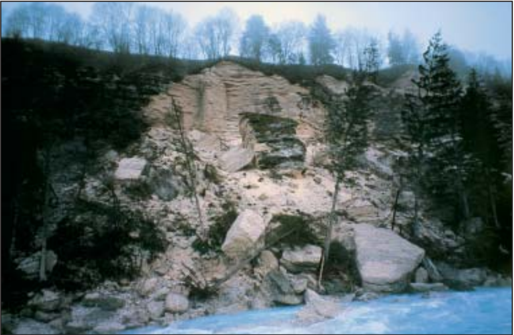
Figure 2: Rockfall in the conglomerate on the right bank of the Soča River near Čezsoča, which occurred during the earthquake on April 12, 1998 (photography Matija Zorn).
