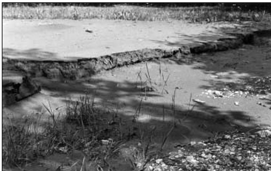
Figure 15: The meadows along the Konjščica were devastated by sand and clay flood material. A view of a layer of flood material, 30 to 50 cm thick, deposited south of Loke settlement.
