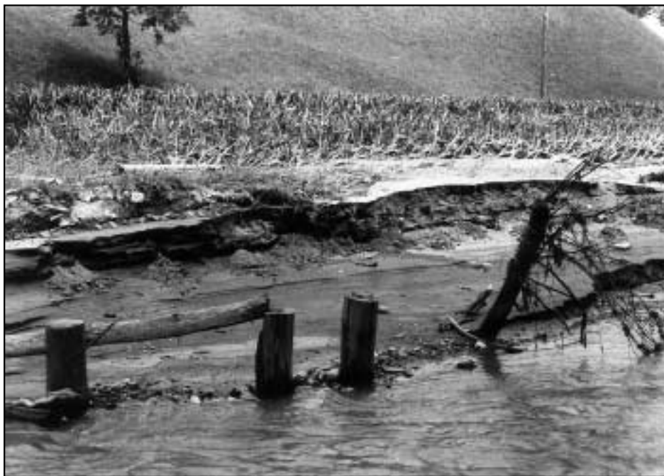
Figure 11: At Loke only a few pilings remained of the village bridge that connected the fields on either side of the torrential Konjščica. In this area, too, the stream »uncontrollably« widened its riverbed and damaged agricultural land.
