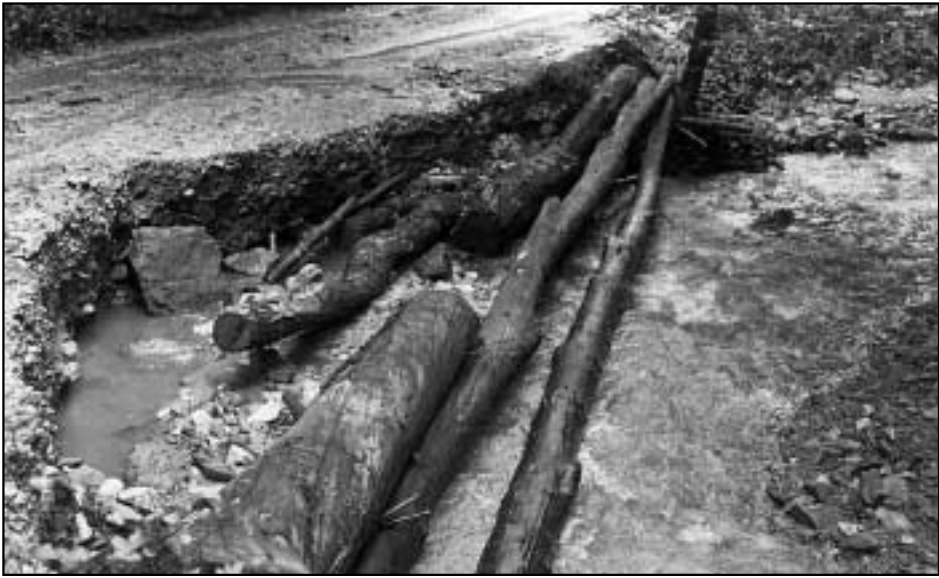
Figure 21: In its catchment area, the Reka (Marija Reka near Prebold) undercut its banks and damaged and washed away the road. Local residents used primitive means to protect the banks from further destruction.
