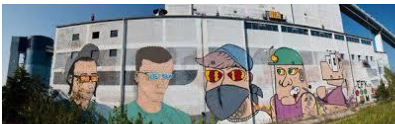
Fig.7: Mural drawn on the old coal separation plant.
