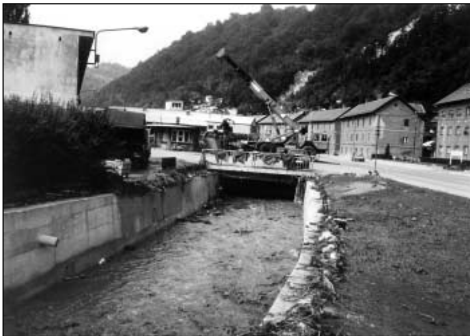
Figure 11: The industrial bridge near one of Trbovlje's factories is a typical example of not considering the natural laws of the fluctuation of streams, since the size of the outlet was greatly underestimated during its construction.
