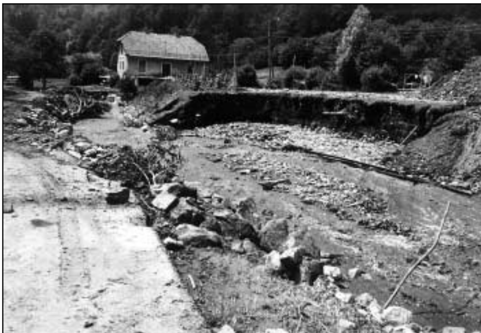
Figure 8: In some places the erosive indentations in the banks along the Kotredeščica were so extensive that they exposed water distribution pipes (on the right).
