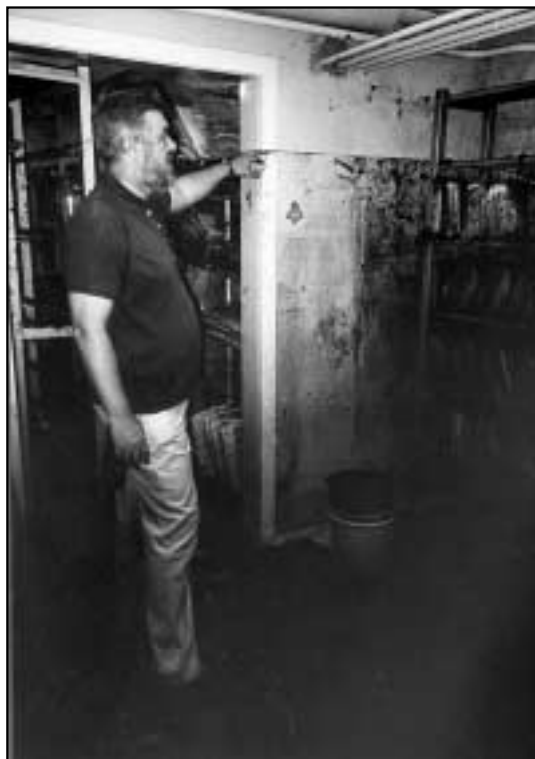
Figure 17: Height of water level in the hospital basement and shelves with ruined archive materials. Slika 17: Višina vode v kletnih prostorih bolnišnice in police z uničenim arhivskim gradivom.
