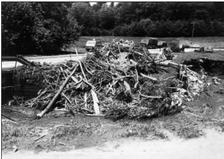
Figure 7: Bridge in one of the settlements on the upper course of the Kotredeščica. Torrential alluvium soon blocked the inadequate outlet, and water flooded all the lower lying part of the settlement.
