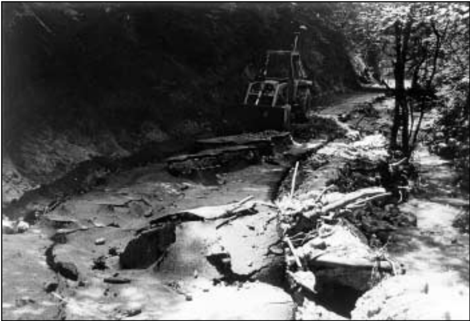
Figure 10: One local road had been paved with asphalt only a few weeks before the storm. In the narrow ravine, the stream and its torrential tributaries cut into the road and completely destroyed it. From the size of the rock debris deposited along the edge of the road, we can see the force of the water.
