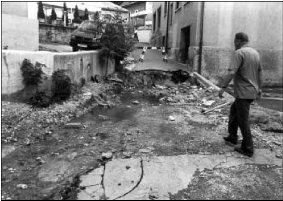
Figure 12: In the center of Trbovlje water came rushing from the mains and spread over the town streets. Part of the roadway was raised and carried away.
