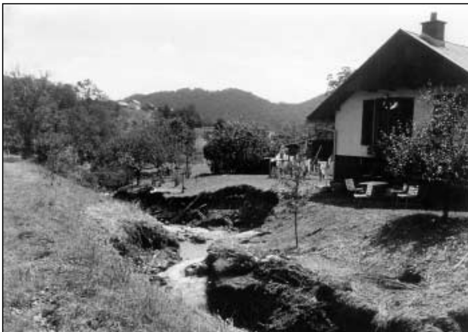
Figure 20: The riverbed of a smaller stream widened and deepened by erosion threatened a house near Litija. How deep the side erosion will be the next time a storm occurs and whether the house will then be far enough from the stream are questions we must answer in dealing with the issue of natural disasters as a whole.
