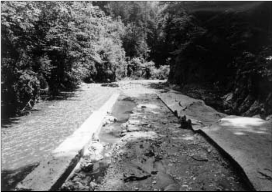
Figure 6: A completely destroyed section of road in the Kotredeščica catchment area. Here the valley narrows completely in limestone, and therefore the power of the water was even greater. The only thing that was remained was a buttress while almost the entire asphalt surface was carried away.
