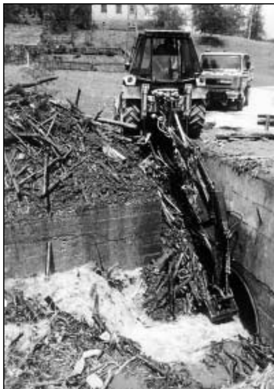
Figure 19: Clearing an outlet in one of the numerous ravines in the surroundings of Litija. Torrential waters mainly carried wood debris among which there was considerable amounts of garbage from uncontrolled refuse dumps along the stream.
