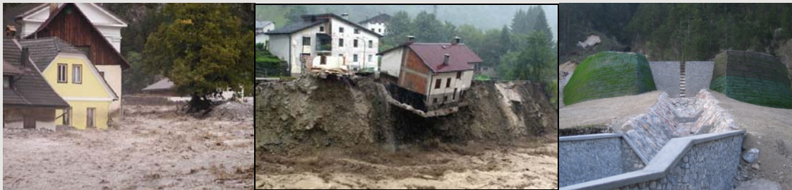
The 2003 flash flood and the risk mitigation works (source: Malborghetto-Valbruna municipality)
