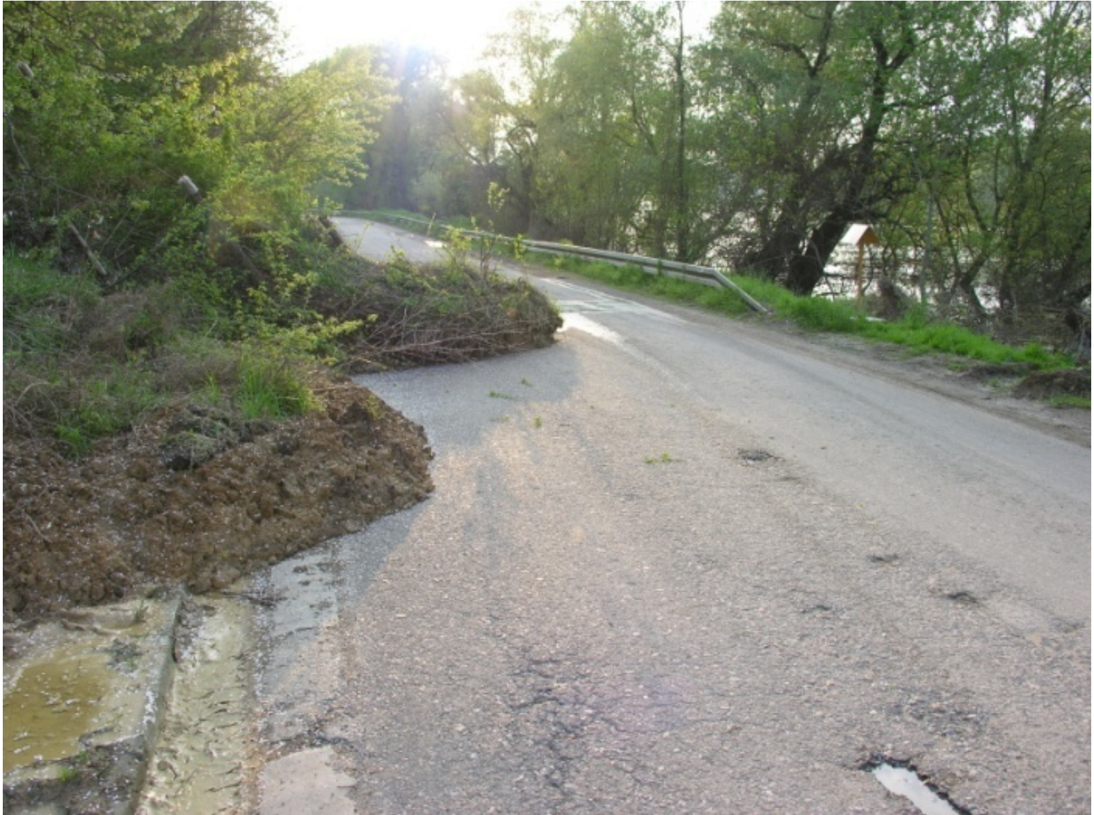
A road obstructed by earth flow near the village of Banoštor (21. 04. 2006. photo: Mészáros M.)
