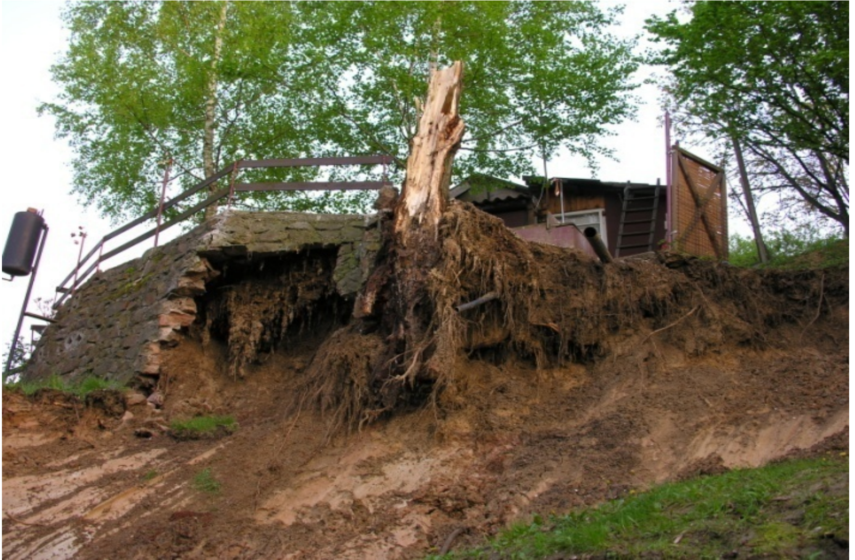
A house damaged by a shallow landslide in the vicinity of Banoštor (21. 04. 2006. photo: Mészáros M.)
