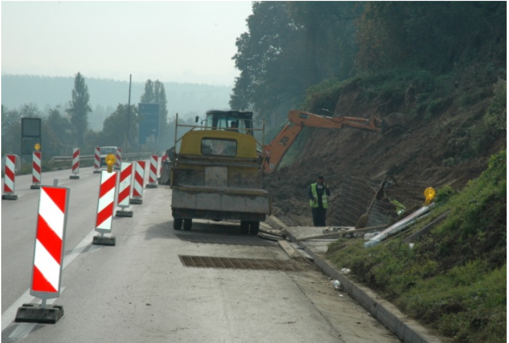
REPAIR OF A ROAD DAMAGED IN SLOPE MOVEMENT NEAR SREMSKI KARLOVCI (2006. 04. 20., Mészáros M.)
