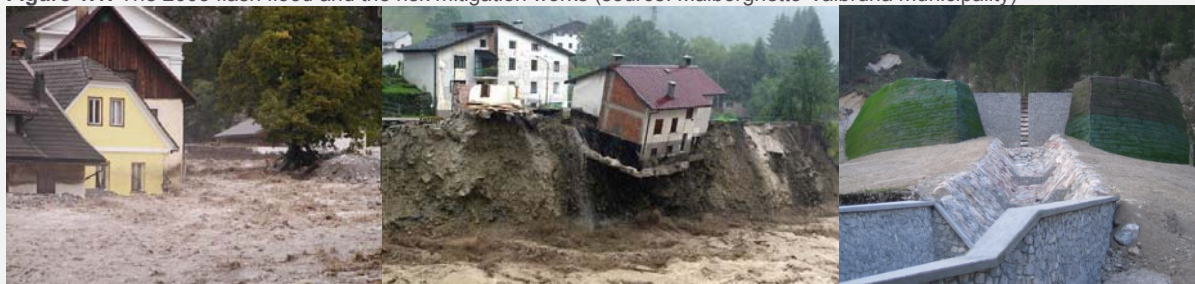
Figure 1.1: The 2003 flash flood and the risk mitigation works (source: Malborghetto-Valbruna municipality)
