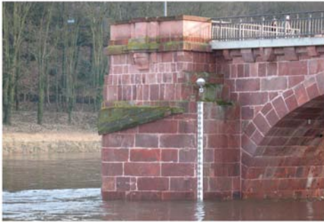
Figure 8: Water gauge at ruins of Pöppelmann Bridge in Grimma
