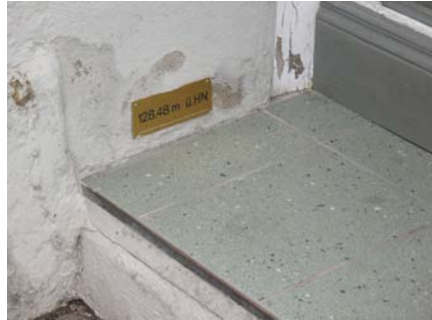
Figure 9: Altitude sign of private threshold (indicating its position 5.12 m above the normal river altitude of 123.36 meters)
