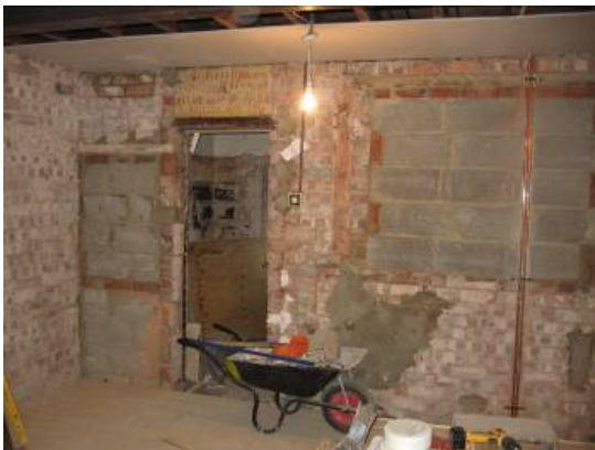
Figure 6: A 'stripped out' house
