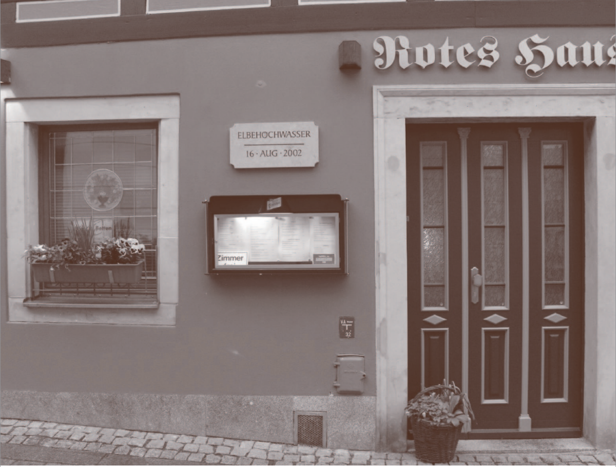
08 Flood marker in Bad Schandau, Germany (2009)
